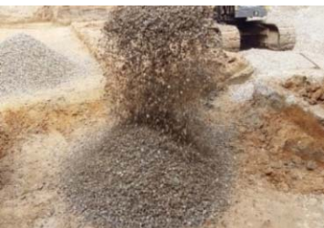
5. Mixing puzzle soils (with 2~3 different sized soils)
