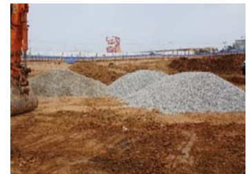
4. Deliver puzzle soils (crushed stones) to site
