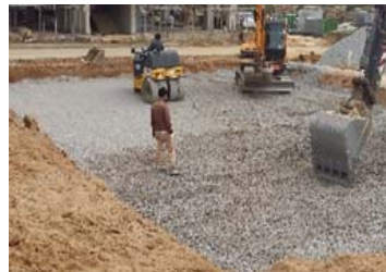
6. Spreading & compaction
